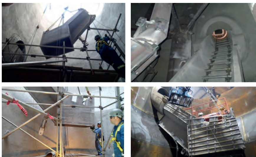
Figure 9 Installation of spent catalyst distributor
